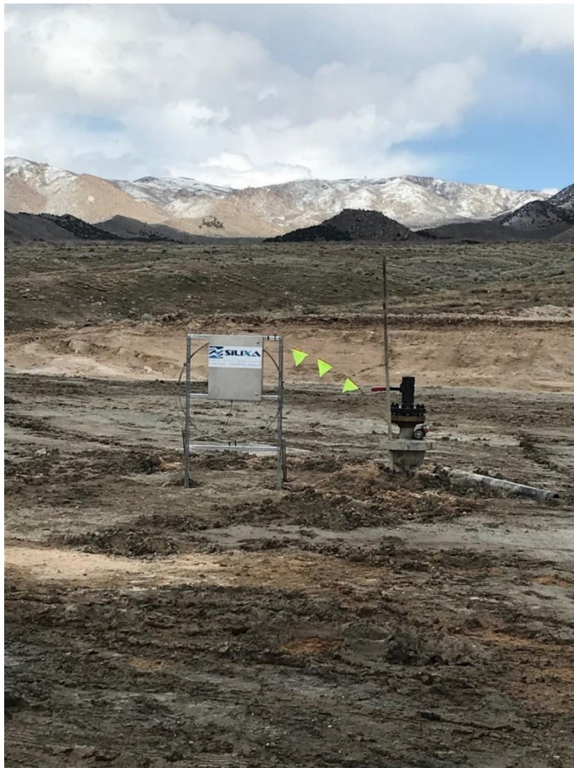
Figure 4: Completed 78-32 wellbore with fiber optic cable at surface.
